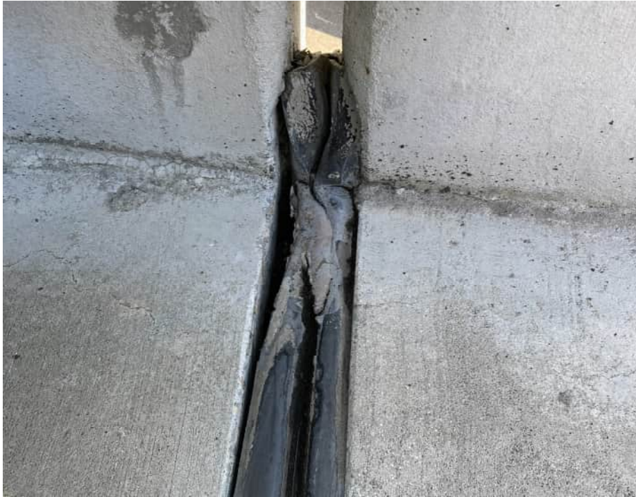
Joint Seal at Bent 9
