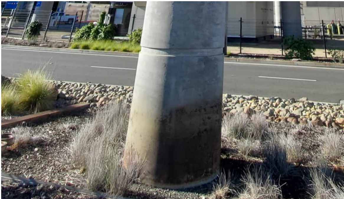
Sprinkler Staining on Columns at Terminal End
