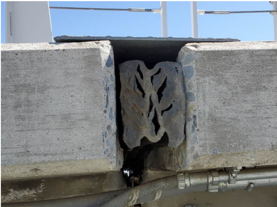
Joint Seal at Bent 9
