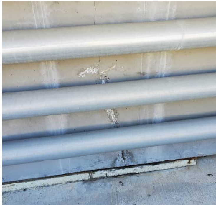
Cracking over Bent 12 Viewed from Track
