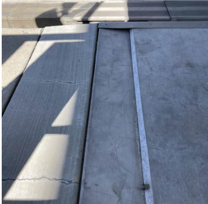
Concrete over Joint at Concourse End
