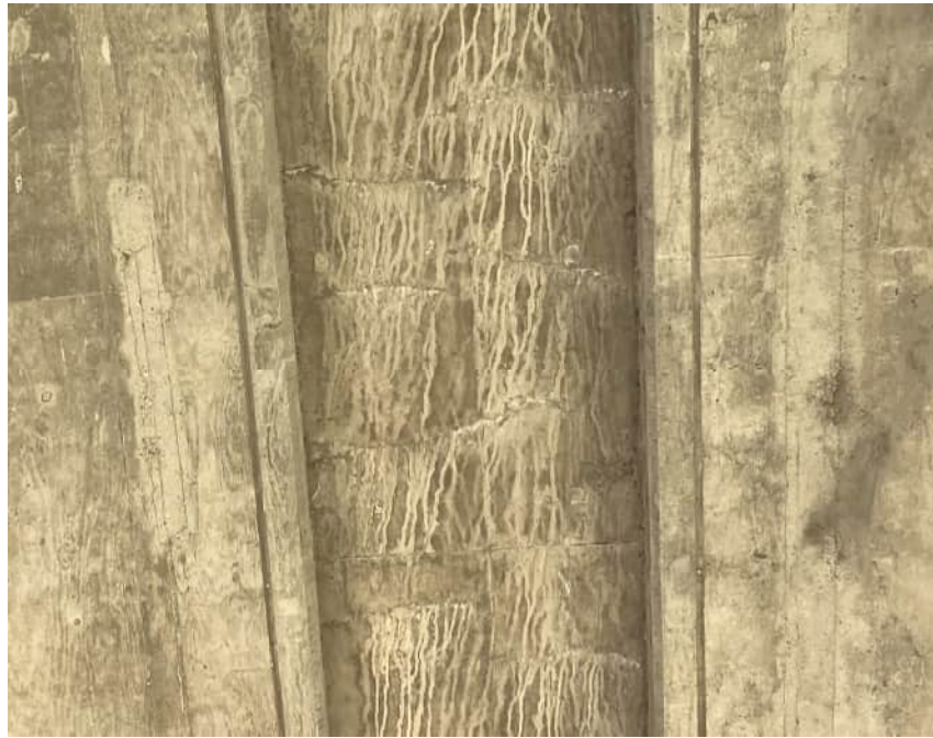
Pattern Transverse Cracking & Efflorescence in Spans 4 - 9
