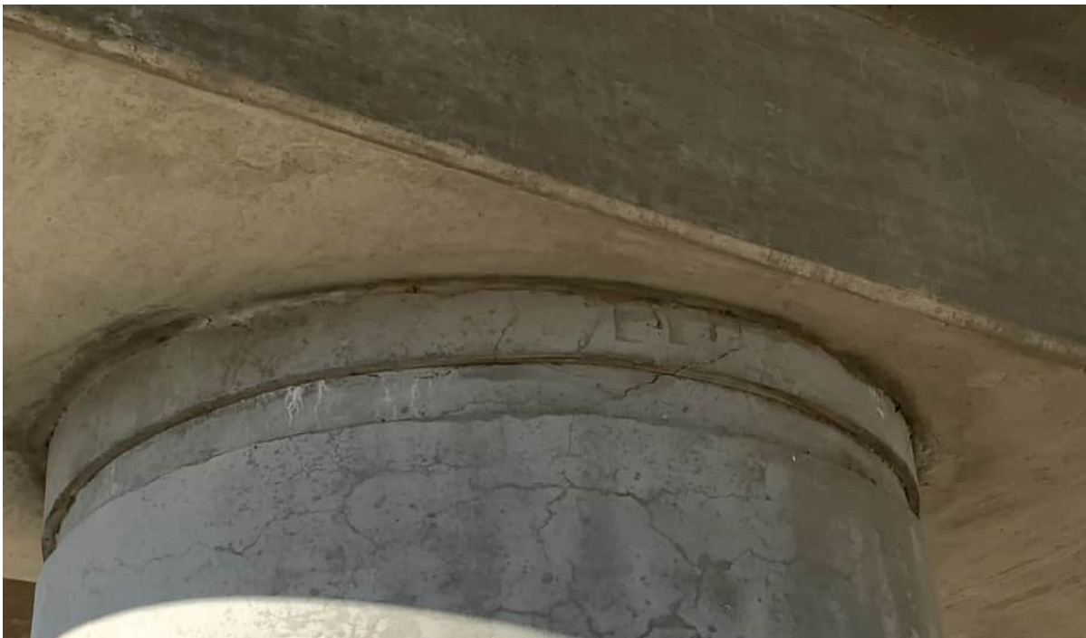
Column Cracking Bent 10 East Column
