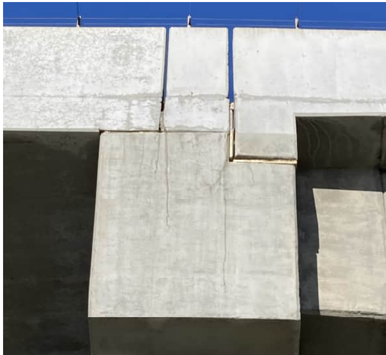
Crack at corbel Bent 4
