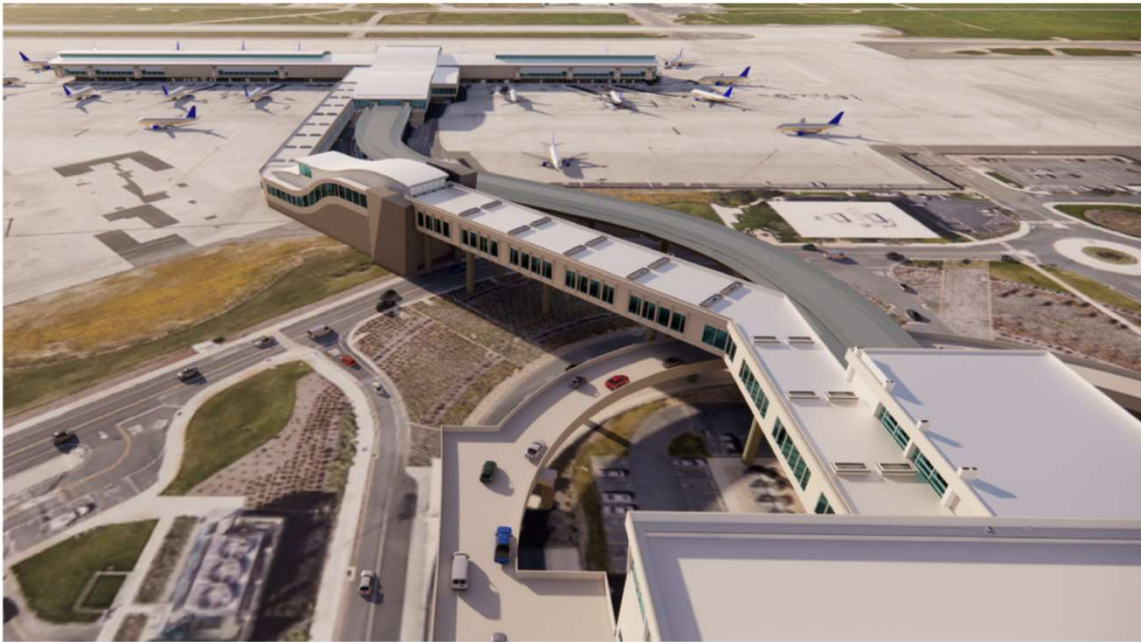
Overhead View of Walkway from Terminal B
